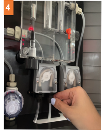
4 Screw in the connector
