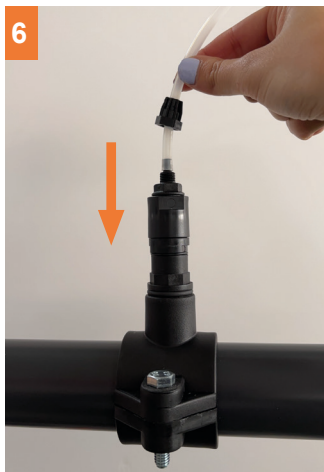
6 Push the rigid tubing along with its connector into the injector.
