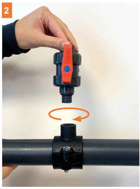
2 Screw the valve into the sleeve, following the order of components from F to D.
