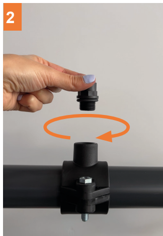
2 Screw the adapter into the sleeve.
