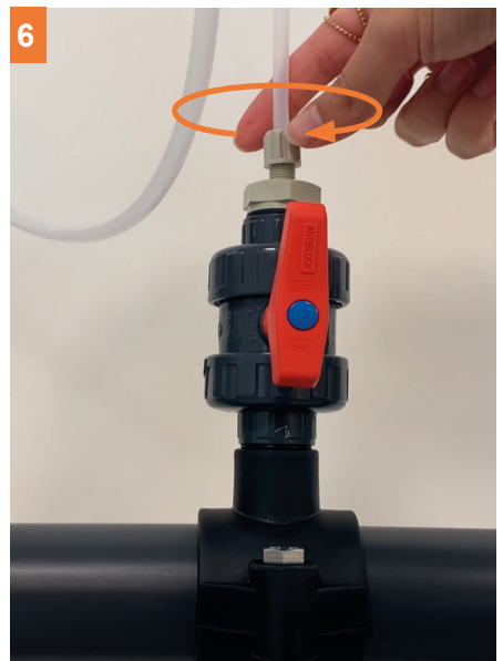
6 Screw in the connector and check that it has been tightened correctly.
