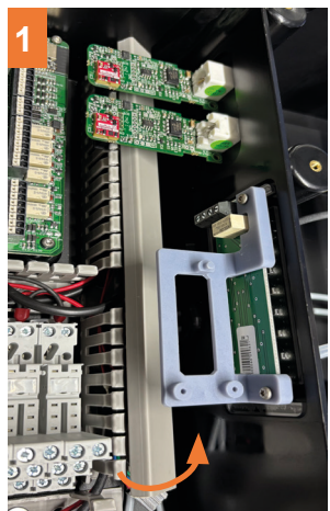
1 Open cable channel to access the VSP cable
