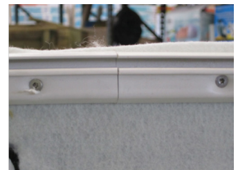
• Installing the slats on a single panel
