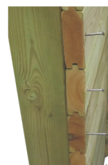
Attach reinforcement one screw each with per board
