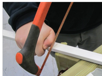
• Trimming the liner profile
