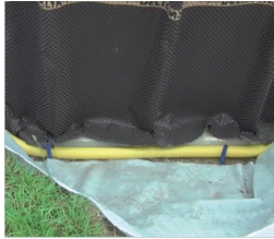
Perimeter drainage
