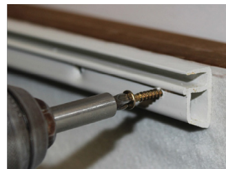
• Securing the liner profile
